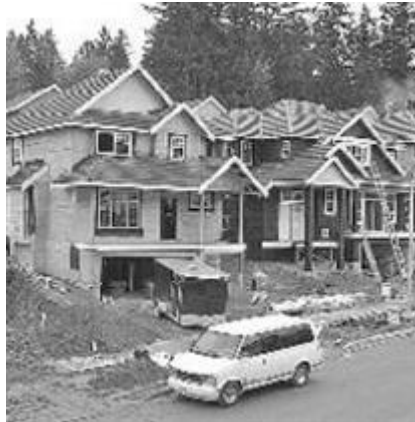
CREDIT: Peter Battistoni, Vancouver Sun In some areas, the cost of the land itself accounts for close to half the total cost of housing units built on it
